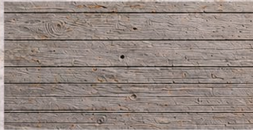
3 BOARD-FORM CONCRETE EXTERIOR
